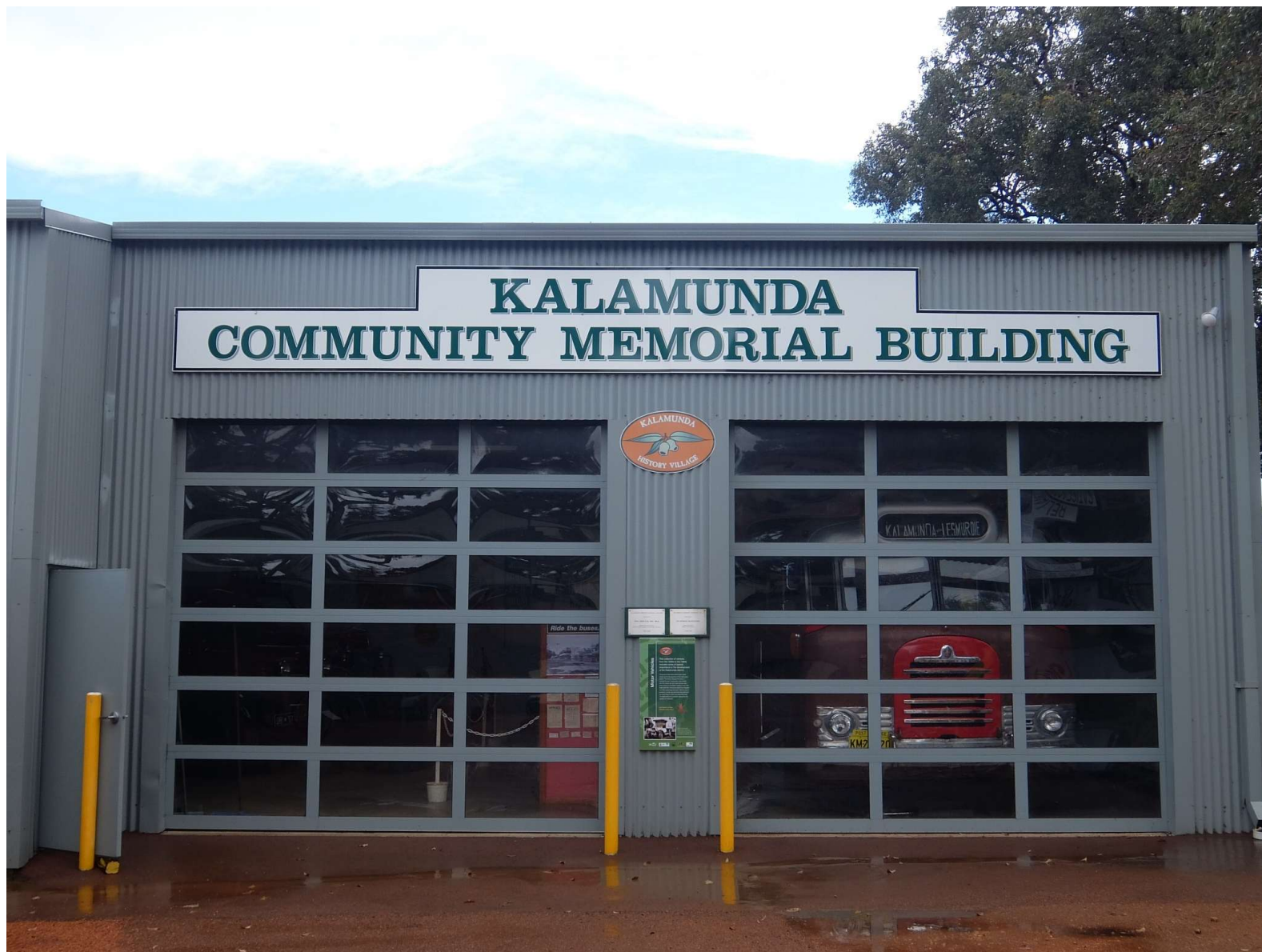
Memorial Building with Pat's Bus
