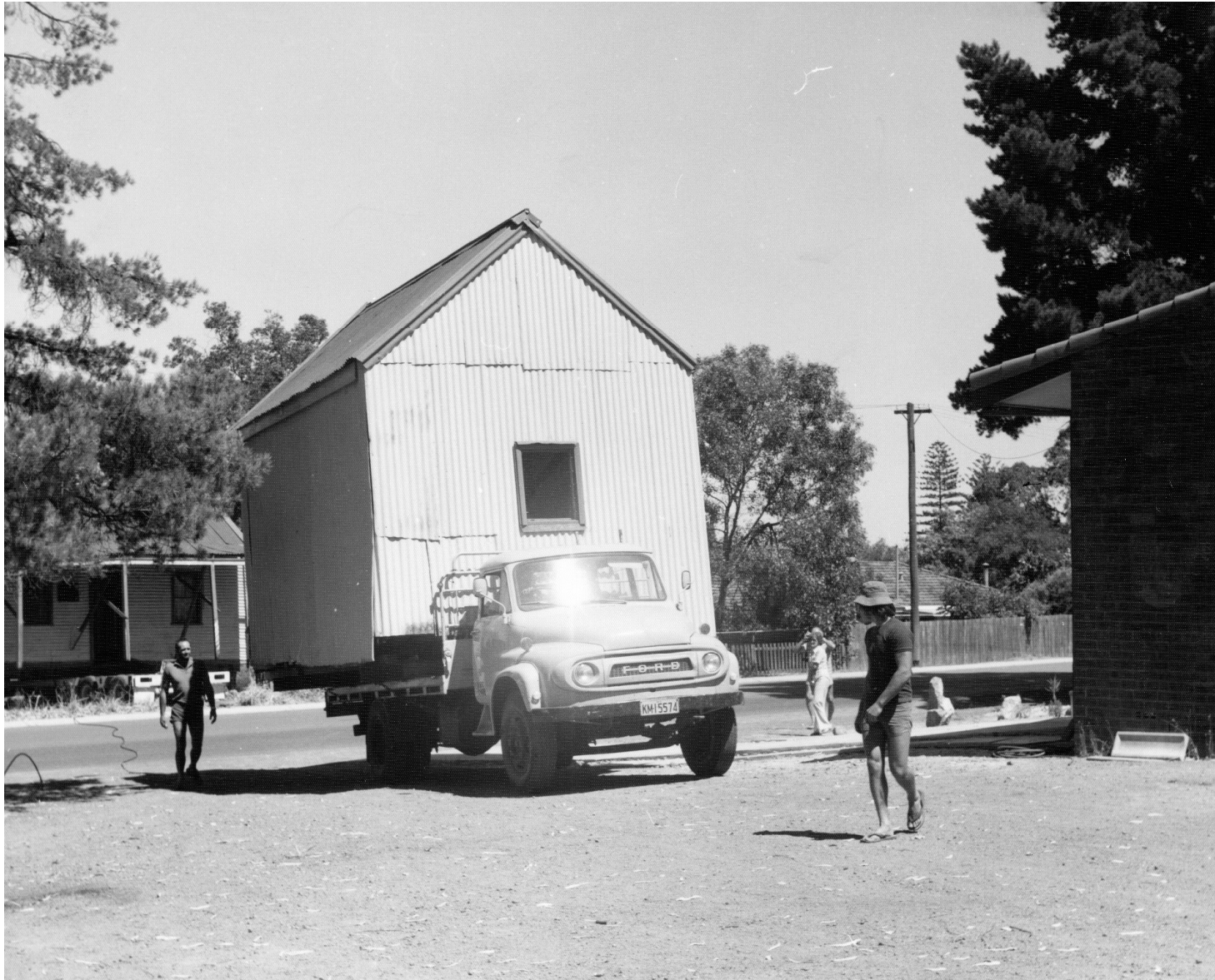
Moving the original McCullough Cottage post office building
